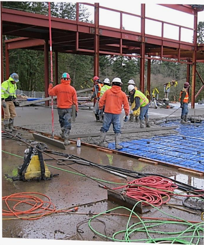
Columbia West conducting concrete testing at Woodburn Elementary School.
