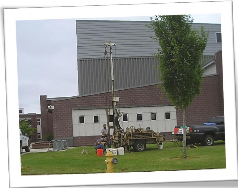
Columbia West conducted a geotechnical investigation at Camas High School.
